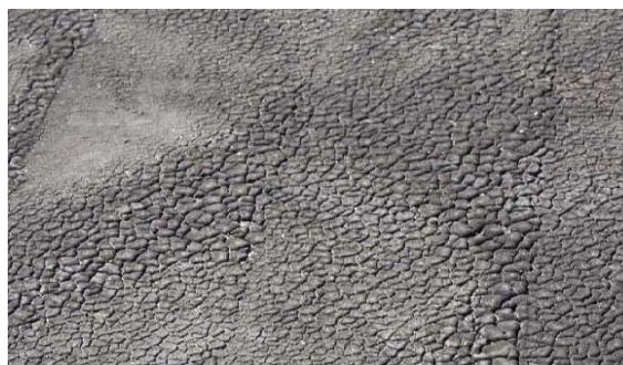
Alligating of BUR Roof
