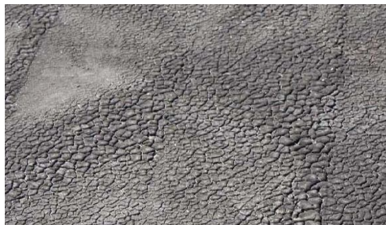
Alligating of BUR Roof
